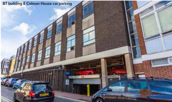
BT building & Colman House car parking
